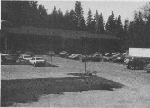
Sierra's current building is nestled amidst the pines of Oakhurst, California, at the southern gate of Yosemite National Park, the second largest national park in the United States.
