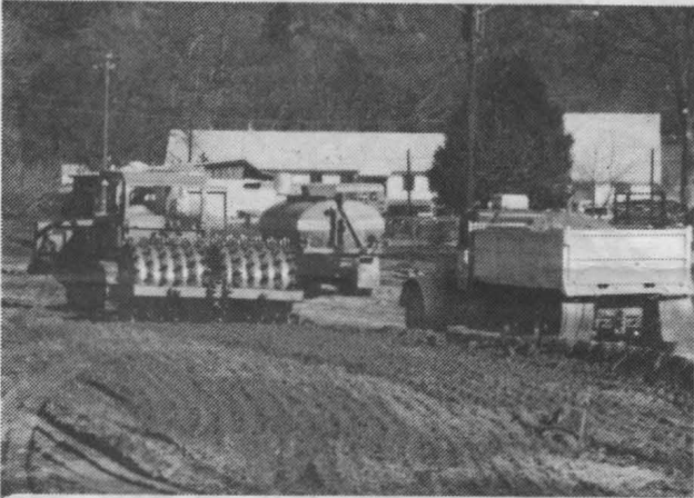
Day 1. Groundbreaking begins! The heavy machinery arrives and ground leveling starts.
